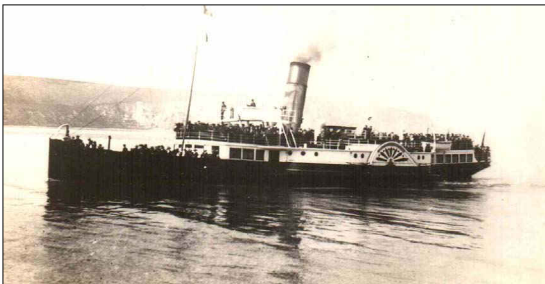
Photograph after 1911 when "Stirling Castle" had her bridge moved forward of the funnel
